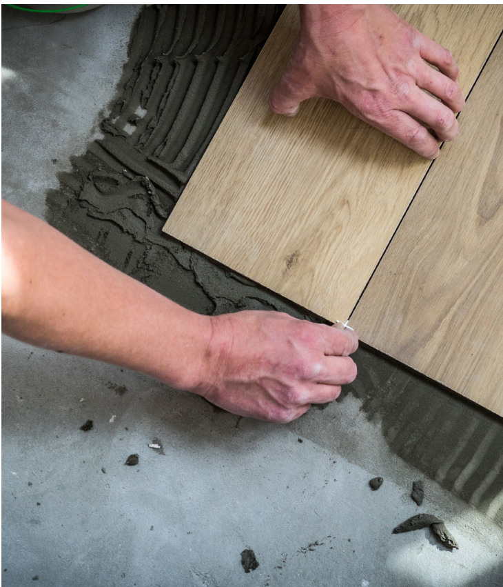
FLOORING INSTALLER FALLS UNDER NATIONAL OCCUPATION CLASSIFICATION (NOC) CODE #7295/73113
