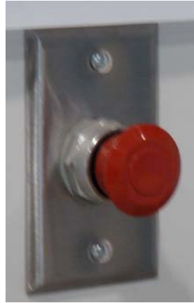
Eye wash safety station emergency power control
