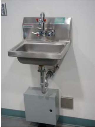
Eye wash safety station emergency power control
